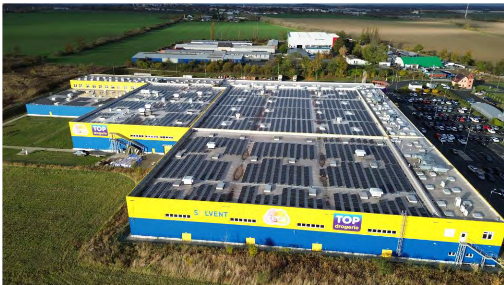
Šetajovice 993 kWp (792 kWac) FVP Lepton 460Wp, Invertoy HUAWEI 40KTL
