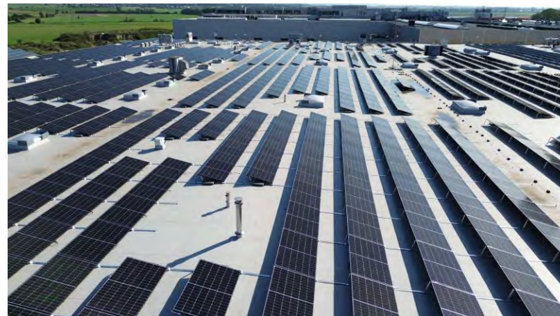
Olomouc 889 kWp (814 kWac) FVP Lepton 460Wp, Invertory HUAWEI 40KTL
