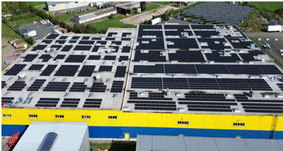
Olomouc 889 kWp (814 kWac) FVP Lepton 460Wp, Invertory HUAWEI 40KTL
