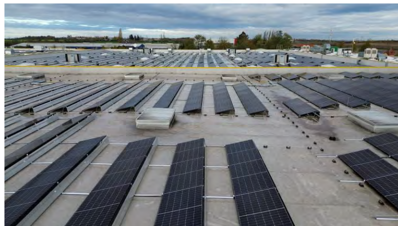
Šetajovice 993 kWp (792 kWac) FVP Lepton 460Wp, Invertoy HUAWEI 40KTL
